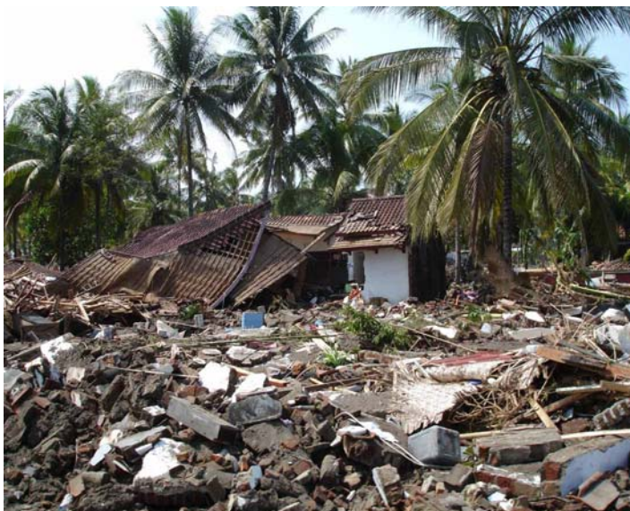
Houses along the coastline were swept away by the tsunami
