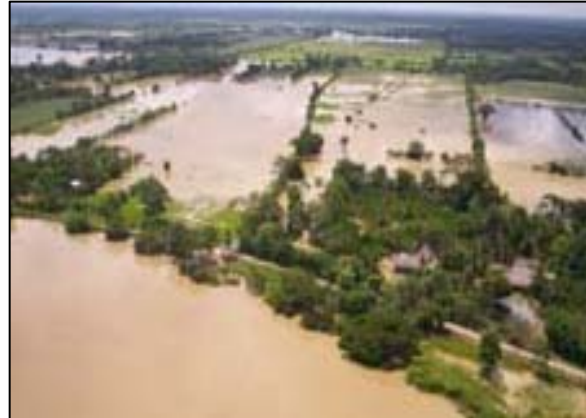
Burst of the Sinú river banks in Córdoba July 2007. Source: CRC??
