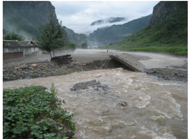
Road destruction in Sinphyong area (International Federation/Aug 2007)
