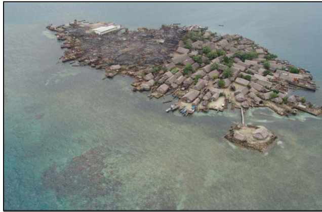
Fire has severely affected the island of Miria Ubgigandu
