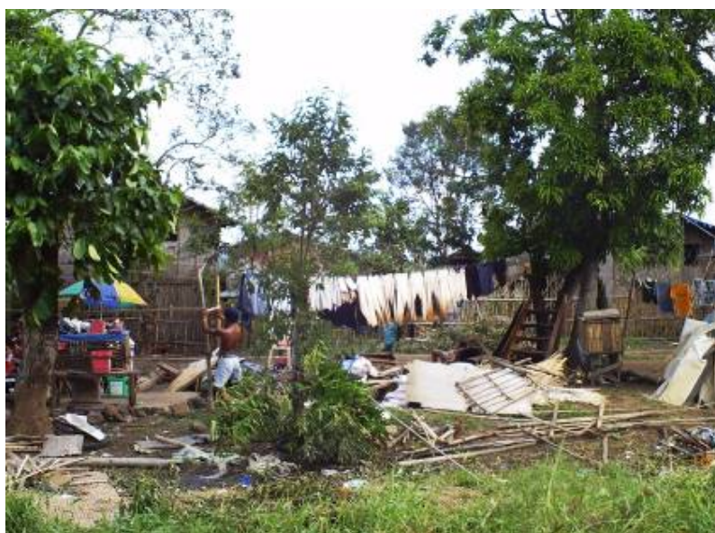
Everyday living resumes and undertaking of repairs to the damage caused has begun. Photo: Alexander Mikadze/ IFRC
