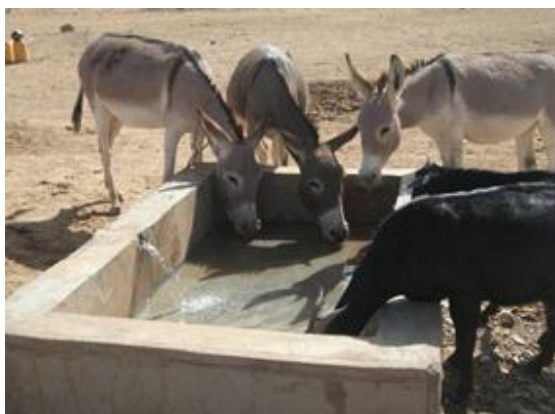
A concrete basin constructed for the watering of livestock in the Brakna region. Photo: IFRC/MRCS
