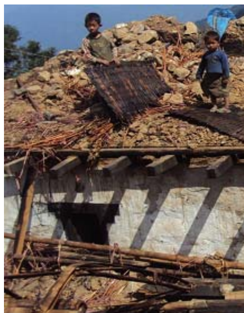
Houses damaged by the earthquake in Pachthar district. Photo: NRCS.
