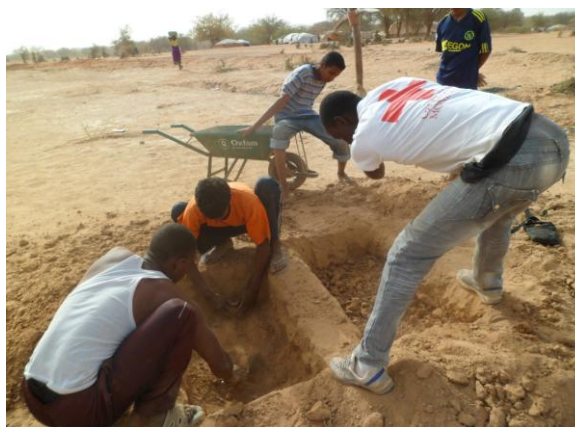
Latrine construction for use by refugee families in Férério Photo: IFRC/BRCS
