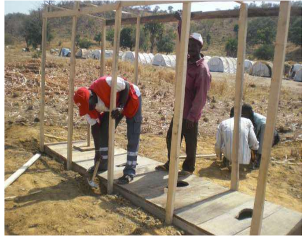
Emergency latrines construction
