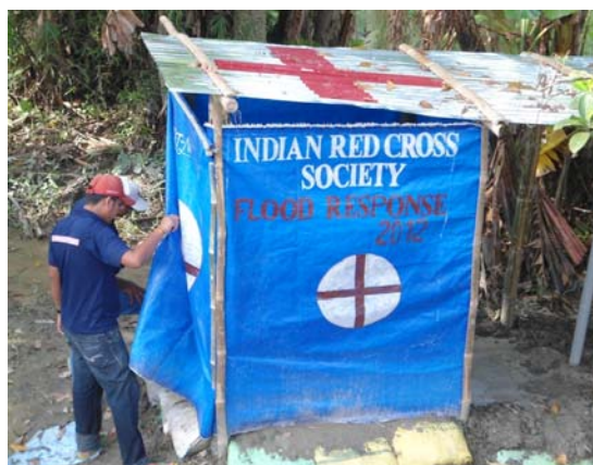
Toilets constructed for the displaced population due to floods in Assam. Photo: Indian Red Cross Society.
