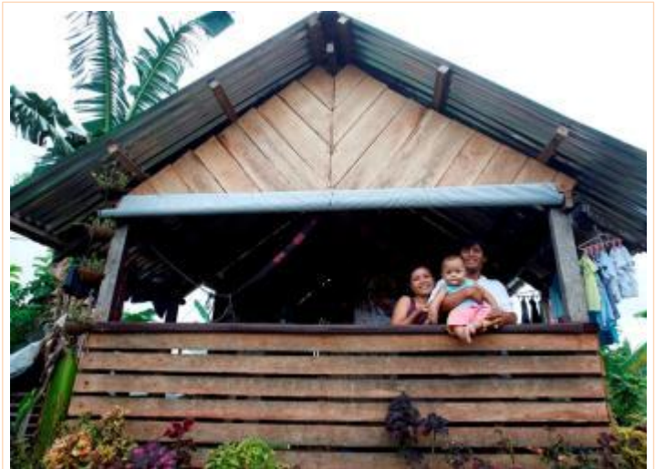
This family received shelter repair assistance from the Red Cross, seen here inside their repaired house at Barangay San Rafael in Cateel, Davao Oriental. One year after Typhoon Bopha, the Red Cross Red Crescent continues provide shelter assistance to affected families. Photo: Cheryl Galagalac / IFRC
