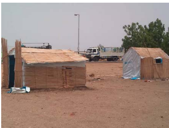
Photo by SRCS: Model emergency temporary shelters constructed by SRCS volunteers during Shelter training
