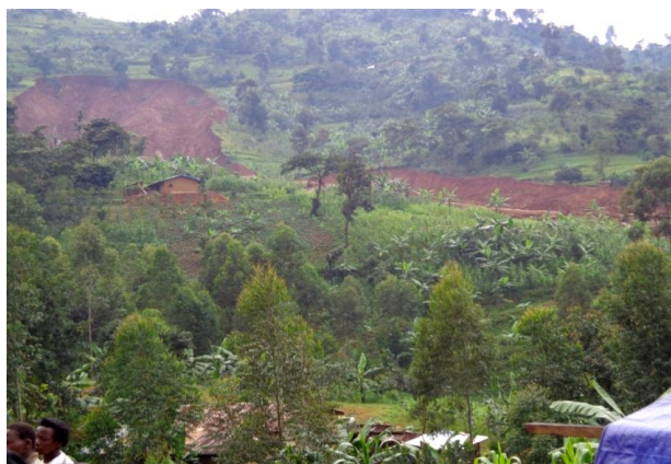
The affected area of landslide which covered 5 acres of land /Photo Uganda RC
