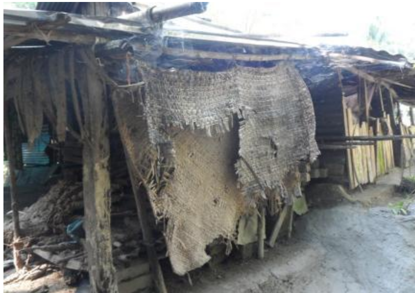
Partially damaged shelters repaired after cyclone Mahasen. Photo: IFRC.
