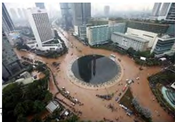
Floodwaters inundate the Hotel Indonesia traffic circle in Central Jakarta in January 2013. (Source: The Jakarta Globe , 16 January 2013)
