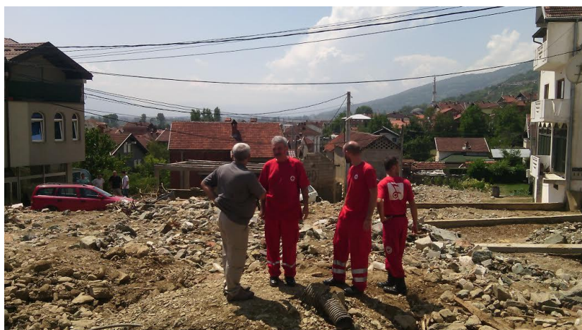
Needs assessment over a collapsed building.
