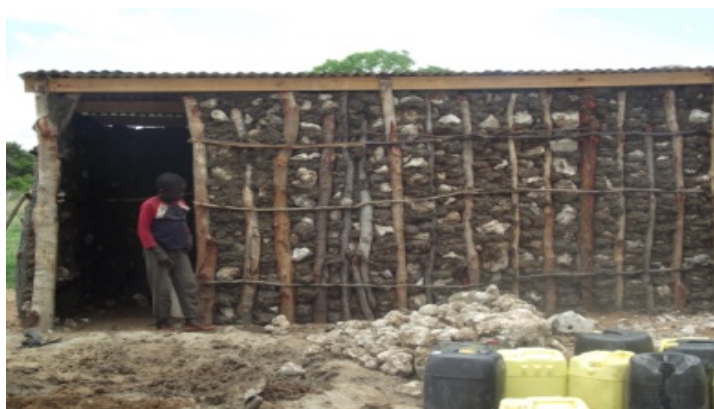
A complete shelter for OVC and family. Photo: NRCS
