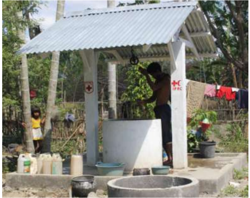
New well in Bitirai, Manufahi district built by CBHFA project
