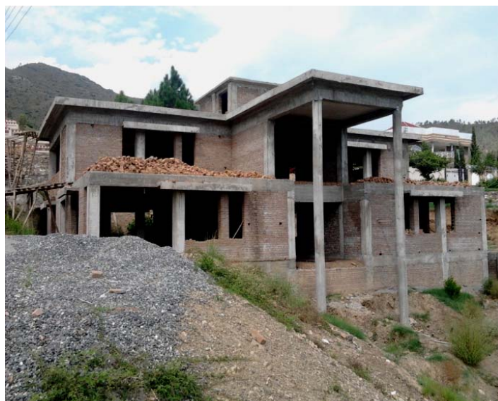
PRCS Swat district branch under construction, KPK province.
