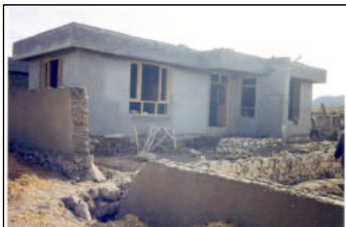
New health clinic under construction
