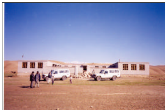
Construction of new school buildings is almost complete
