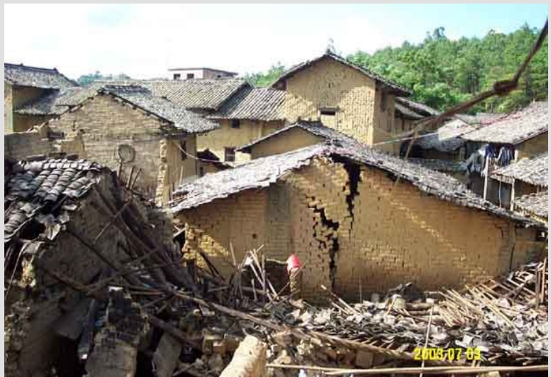
2.16 million homes have been damaged so far due to severe flooding in China.
