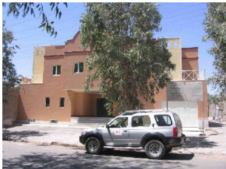
Despite the delay, by the beginning of June 2006, the construction of the UHC was completed
