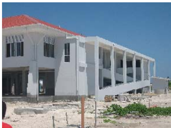
Apart from being functional spaces for communities, the storey buildings can serve as safe havens for people in times of disasters.
