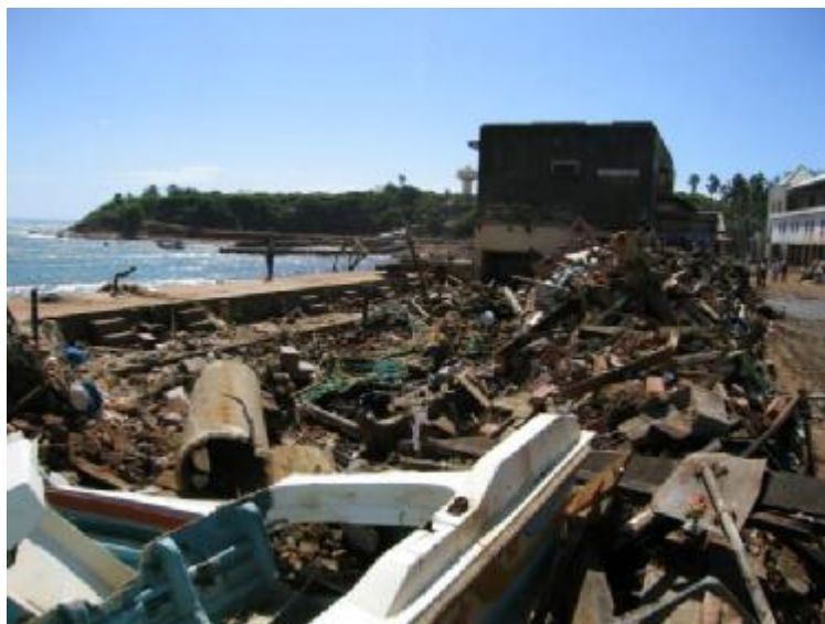
Hambantota: Destroyed houses on the coast
