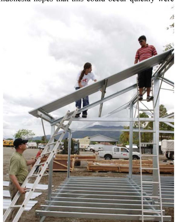
Galvanized steel frames being erected on first batch of the 20,000 transitional shelter units being provided in Indonesia.
