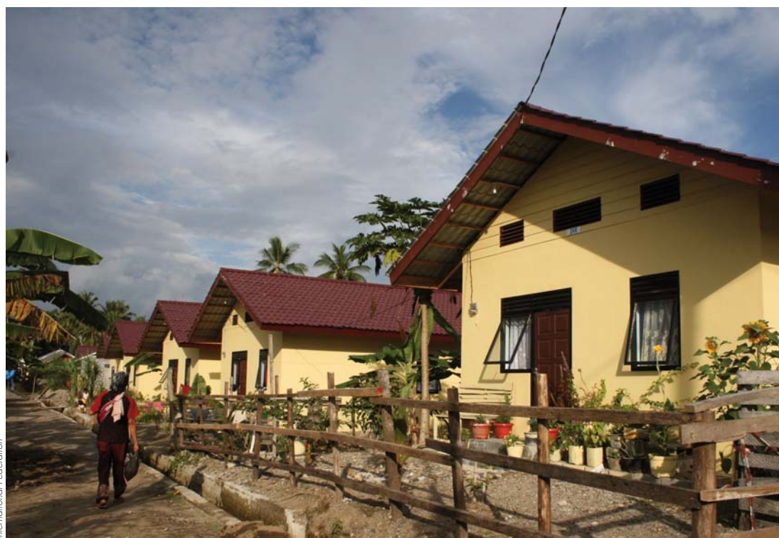
New houses for tsunami survivors built by the Red Cross Red Crescent in Teunom, Aceh Jaya.
