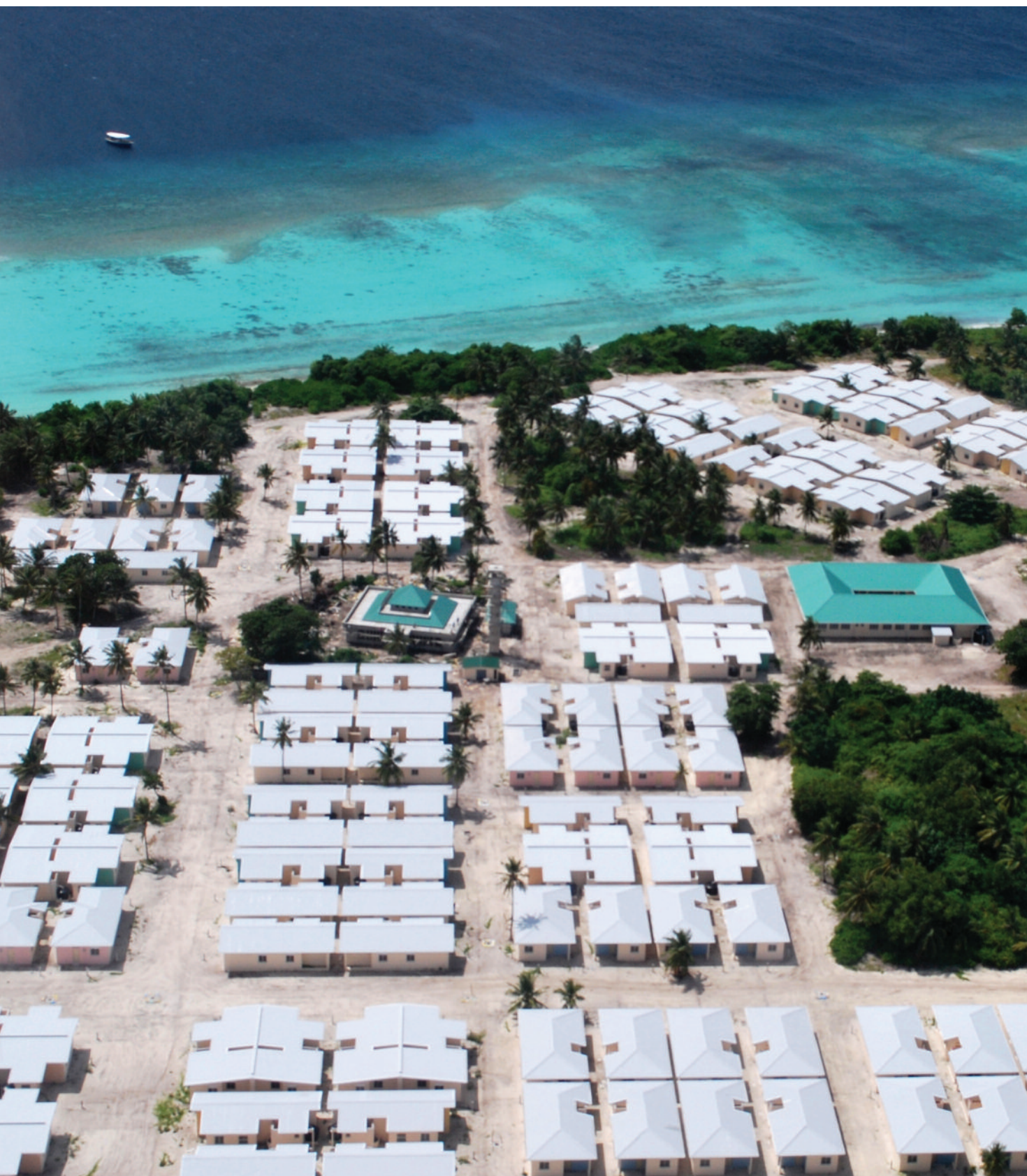
An aerial view of Dhuvafaru, Maldives; houses and community buildings are now complete and ready for handover.
