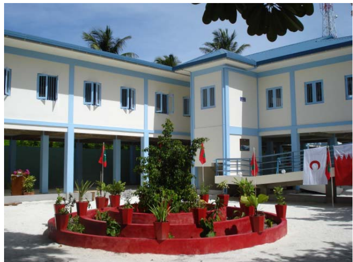
This home for people with special needs is designed to withstand floods and high sea water levels. International Federation/ Valpuri Saarelma.
