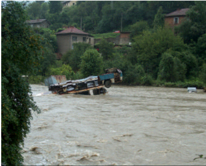
The heavy rains and storms which hit Bulgaria in the end of May 2005 caused damage to buildings and infrastructure of 25 municipalities in the country
