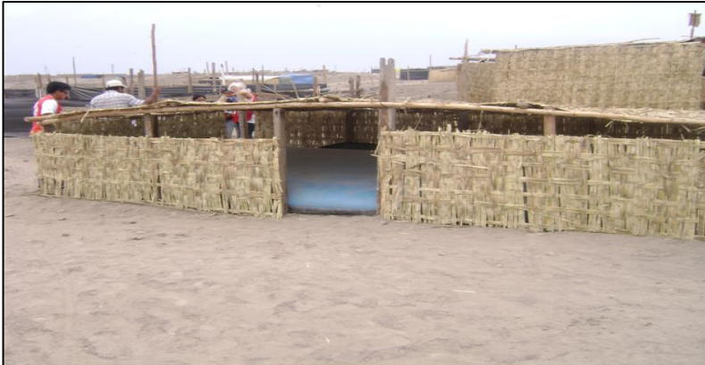
The Nuevo Pisco Association of Affected People in Los Molinos- Pisco organized to build a shelter to protect their donated "bladder" (water storage bag). Source: International Federation of Red Cross and Red Crescent Societies
