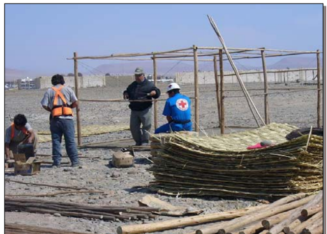
Local materials are used to build PRC Temporary shelters. Source: International Federation of Red Cross and Red Crescent
