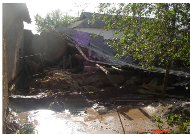
One of the clay houses in the Rudaki district that were destroyed by the mudflow
