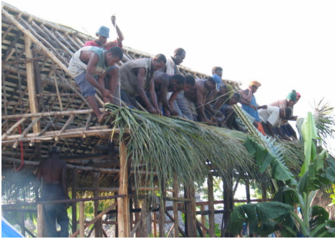
The operation progressed steadily
