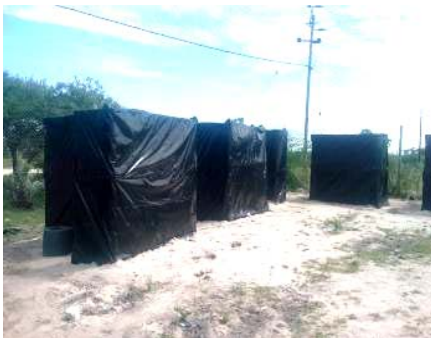
Temporary latrines constructed at Caprivi and Oshikango - Namibia
