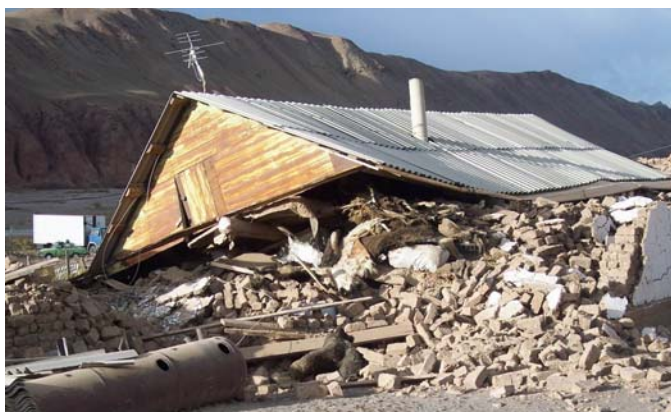
The earthquake leveled Nura village in Alai district.
