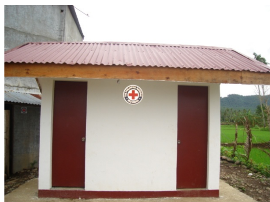
One of the latrines that were constructed in the evacuation camp to cater to the needs of the evacuees (International Federation)
