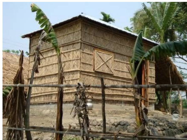
A recently completed core shelter house under the Sidr recovery programme. Photo: Bangladesh Red Crescent Society.
