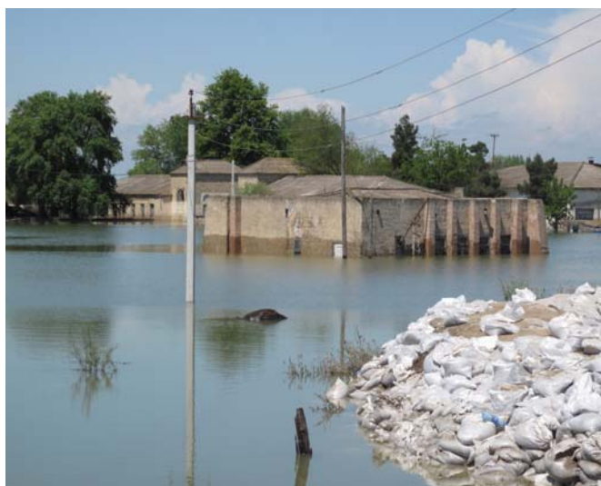
Floods in Sabirabad region with many houses under water and totally destroyed. Photo: Azerbaijan Red Crescent.
