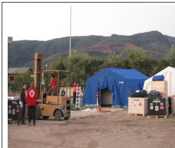
Spanish BCH-ERU installed in Gualañe. Photo source: Gema Arranz/ Spanish Red Cross
