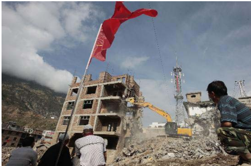
Large machines working in Zhouqu county to pull down dangerous buildings where structure were destroyed by the mudslide. Efforts to clear up the debris and mud is still ongoing. (Photo: Xinhua Net)
