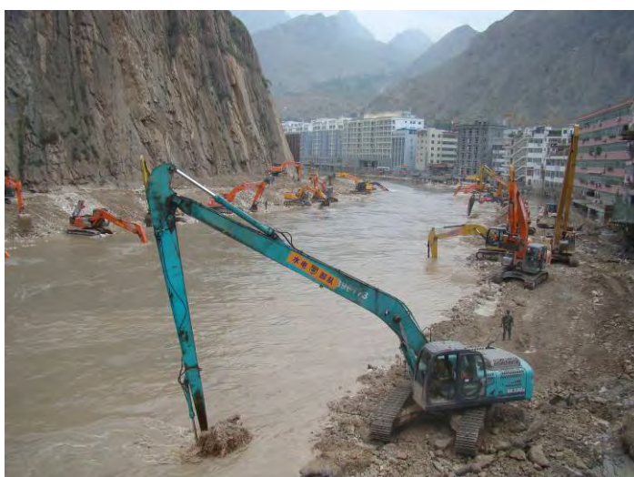
Heavy machineries working alongside Bailong River to clear the barrier lake blocked by tonnes of mud and rocks. Photo: IFRC.
