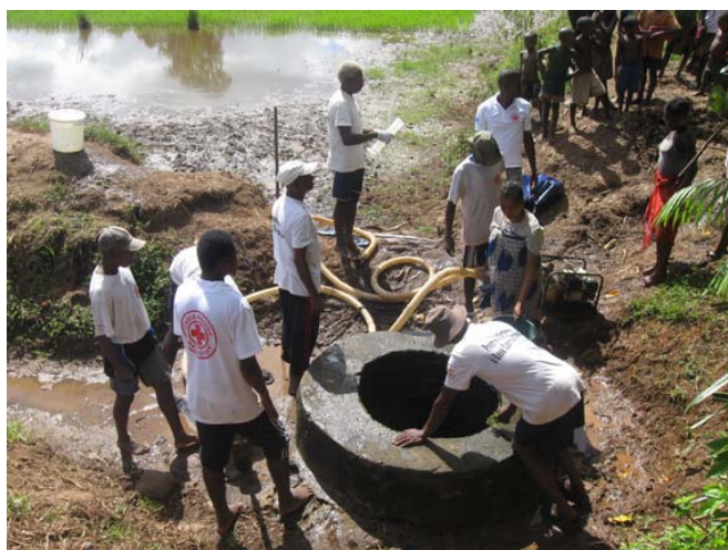
Rehabilitation of wells by MRCS Volunteers Photo: MRCS
