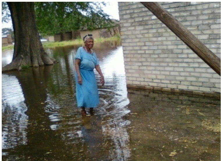
Some of the new infrastructure flooded
