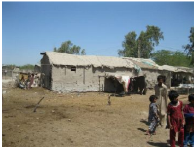
An existing katcha house in Thatta.
