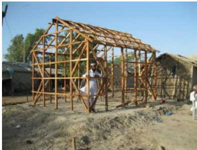
The timber frame under construction.
