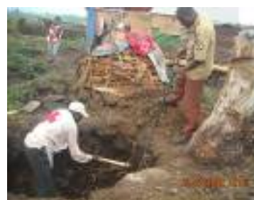
RRCS volunteers constructing a pit latrine: Photo RRCS
