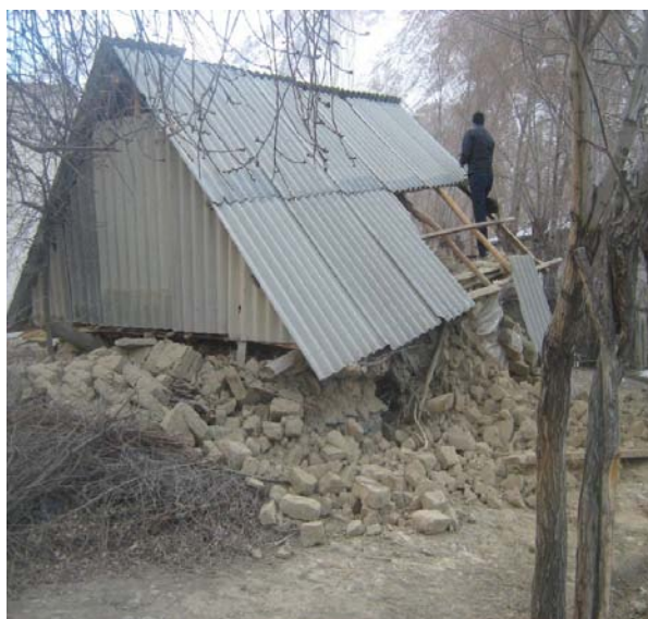
Twenty eight houses were completely destroyed in Gishkhun village, Vanj district
