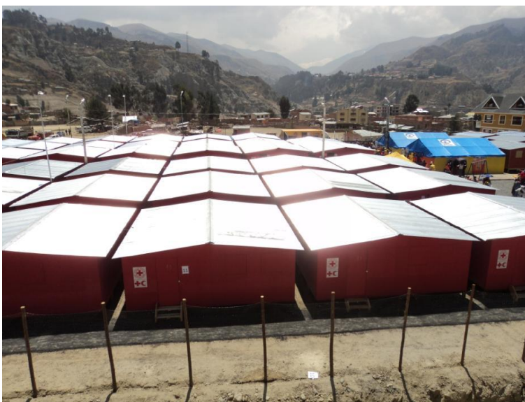
The Bolivian Red Cross constructed 50 transitional shelter modules in Callapa camp to assist 50 families affected by the massive landslide that occurred in La Paz city. Source: BRC
