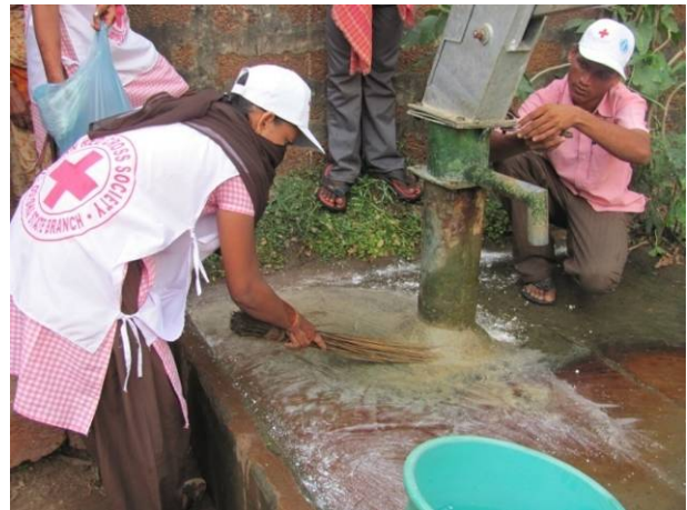
Cleaning of surrounds of water source after disinfecting the same by bleaching powder. Photo: Indian Red Cross Society.
