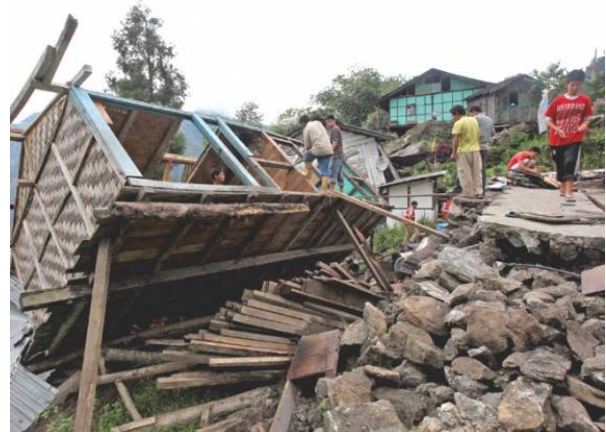
Damaged houses in rural Sikkim. Photo: Indian Red Cross Society.
