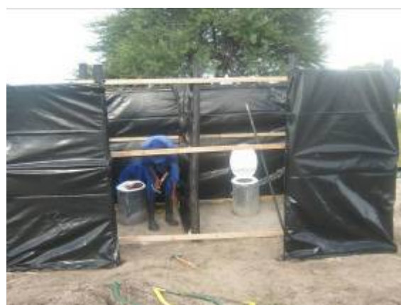
Figure 3: Latrine construction at Oshoopala camp
