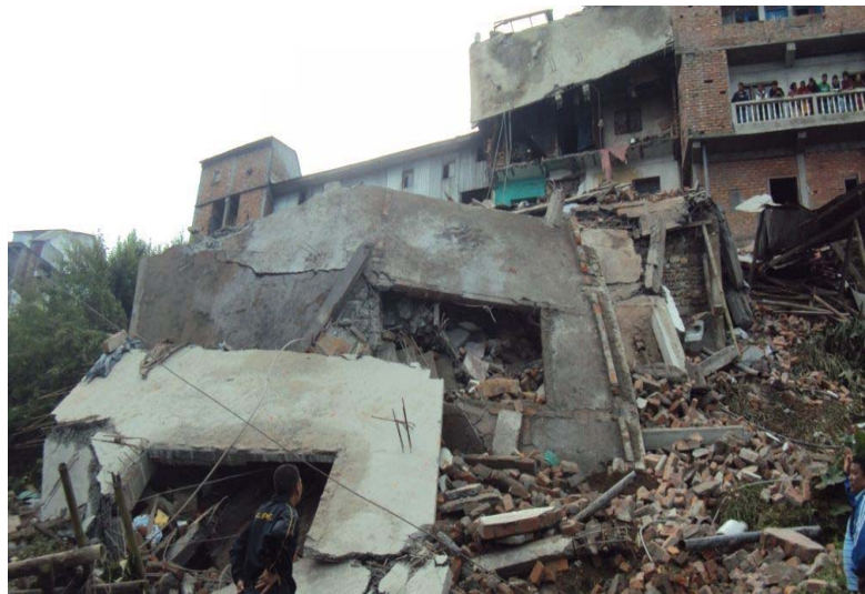
A collapsed building in Dhankuta district. Photo: Nepal Red Cross Society.
